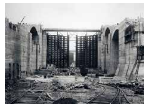
Building of the lock of Panama Canal
