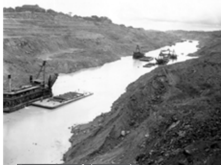
Excavation of the canal
