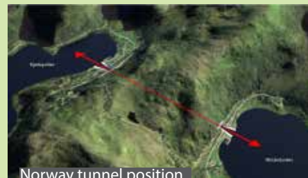
Norway tunnel position
