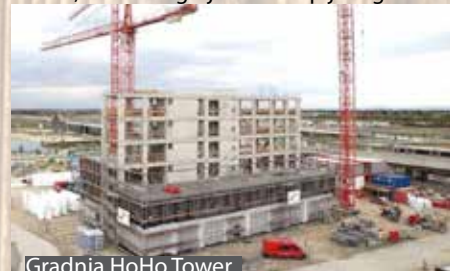
Gradnja HoHo Tower
