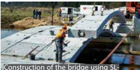
Construction of the bridge using SL-decks with pearl-chain method
