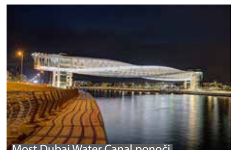
Most Dubai Water Canal ponoči
