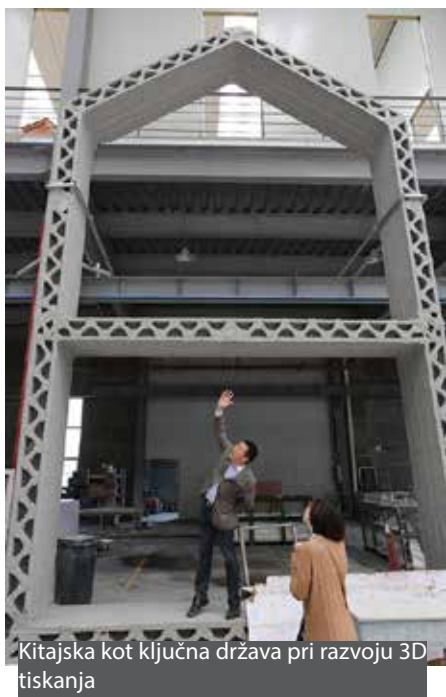
Continuous Concrete Printing – CPP
